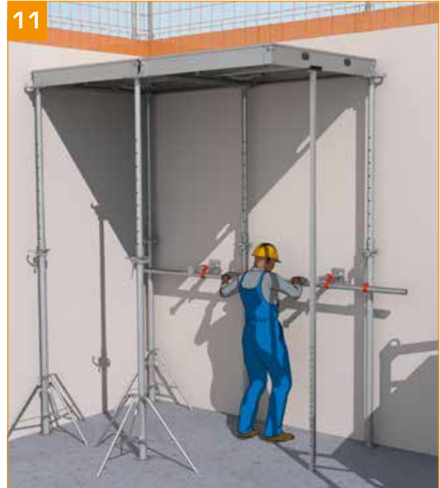
- Set up the final stabilisation of the formwork. - Continue to lay the formwork from one to the next up to the skin.
