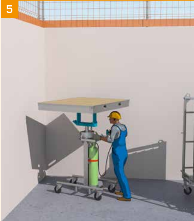
- Move the device to the desired location to start the formwork.
