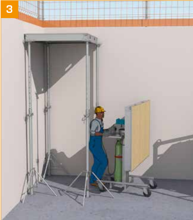
- Position the MaxUp at the desired location, the operator is positioned under the panel fitted previously.
