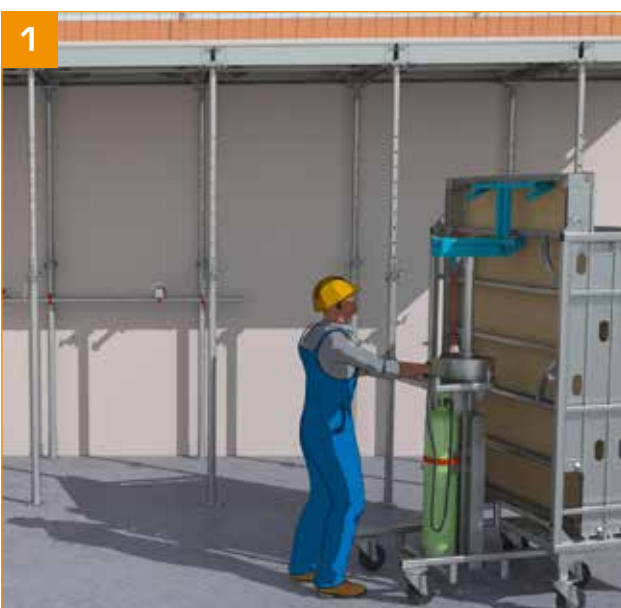
- Retrieve the panel from the rack using the MaxUp and raise it 20 cm to make it easier to move.
