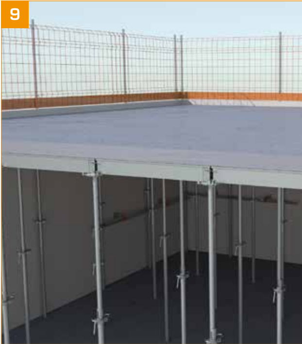
- The cell is formed and the slab is cast.
