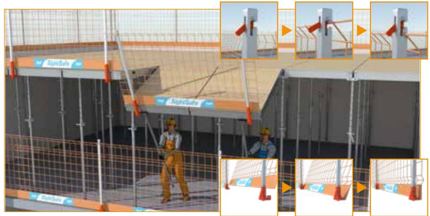
The mesh is locked at the top by the anti-lifting pin and locked in rotation at the base.
