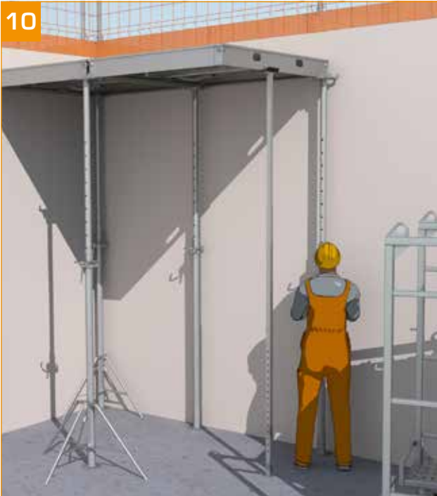
- Position the final 2 props under the panel.
