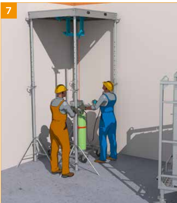
- Place the 4 props with their tripod at the 4 corners of the panel.
