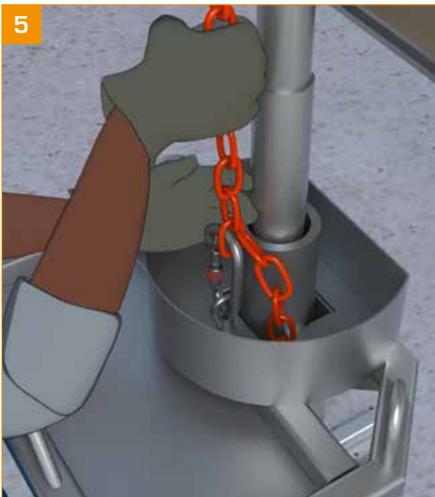
- Secure the chain with the spring hook to maintain the desired height when installing the subsequent panels.
